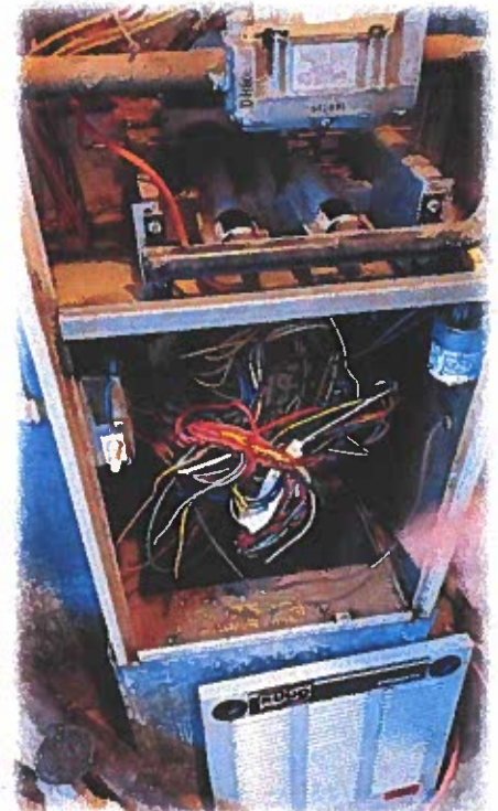
(Furnace in need of replacement)
