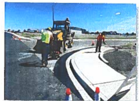
Stover Road Resurfacing
