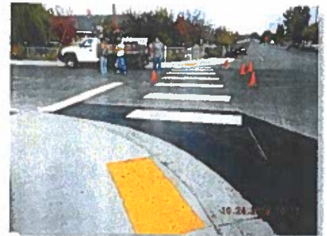
Elm Street and Fir Street Sidewalk Improvements
