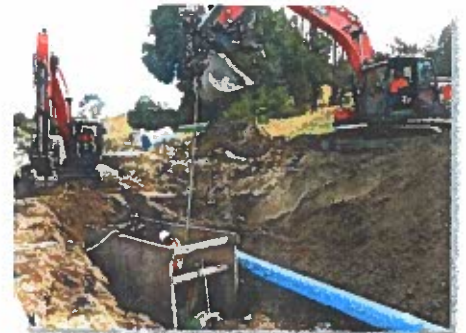
Sanitary Sewer Trunk Main Replacement
