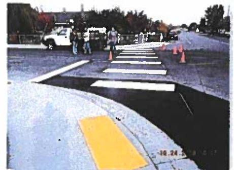
Elm Street and Fir Street Sidewalk Improvements
