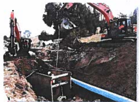
Sanitary Sewer Trunk Main Replacement
