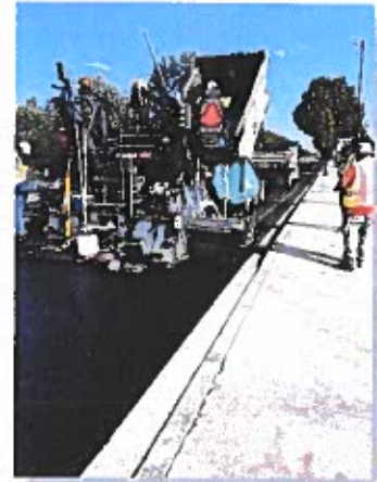
Wine Country Road Resurfacing
