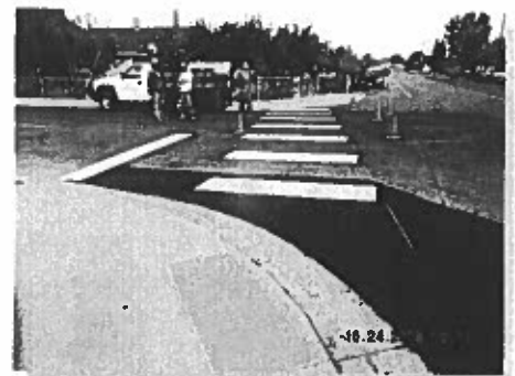
Elm Street and Fir Street Sidewalk Improvements
