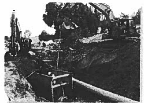
Sanitary Sewer Trunk Main Replacement
