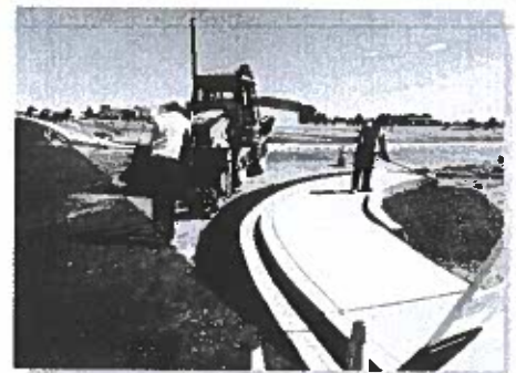
Stover Road Resurfacing
