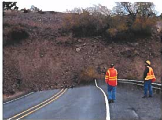
Figure 3.16. Nile Valley Landslide on SR-410 Source: Washington Dept. of Transportation
