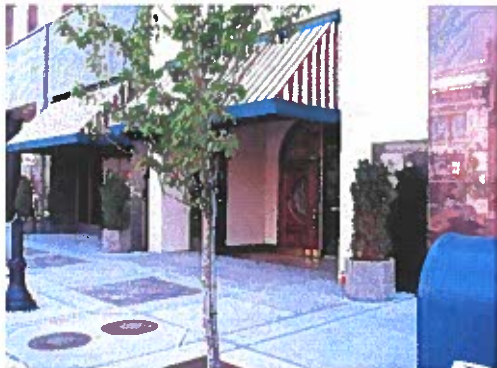
Recess, awning, plantings highlight entrance
