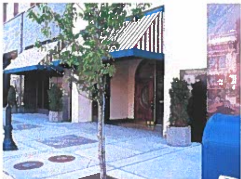
Recess, awning, plantings highlight entrance
