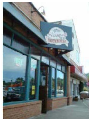
Sign highlights building entrance
