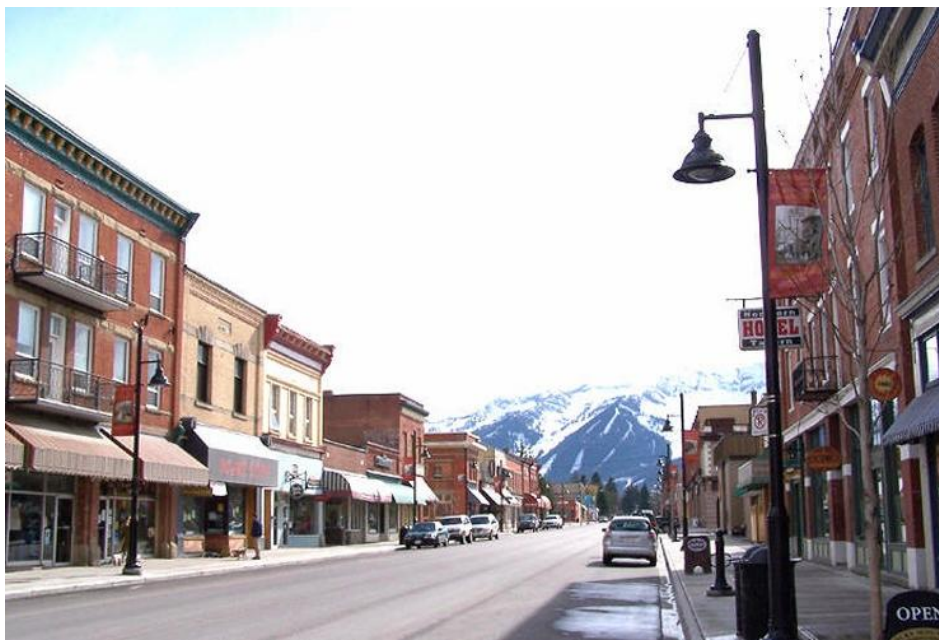
Varying building parapet treatment adds interest to streetscape
