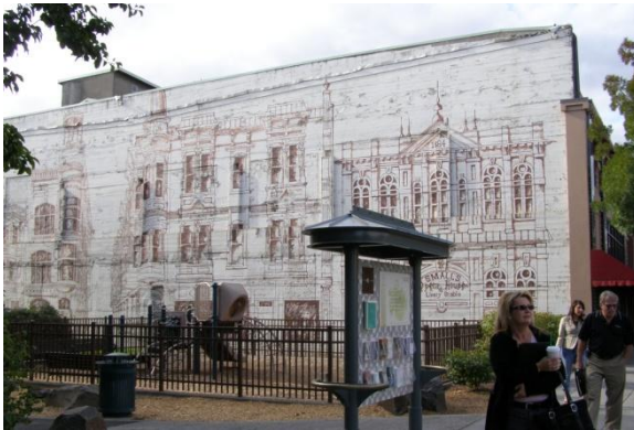
Mural used to screen blank wall
